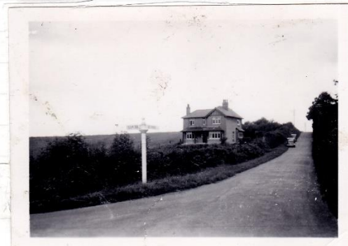
This photograph showing the tram inn road - Belmont junction.
