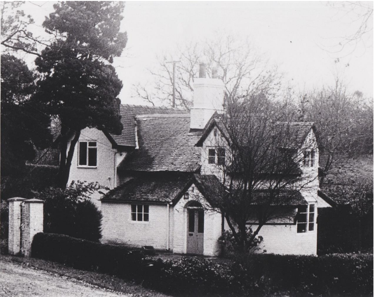
Dewsall Lodge in about the 1950s. Note that part of the pent roof on the right has been removed to allow more light in to the front ground-floor window.
