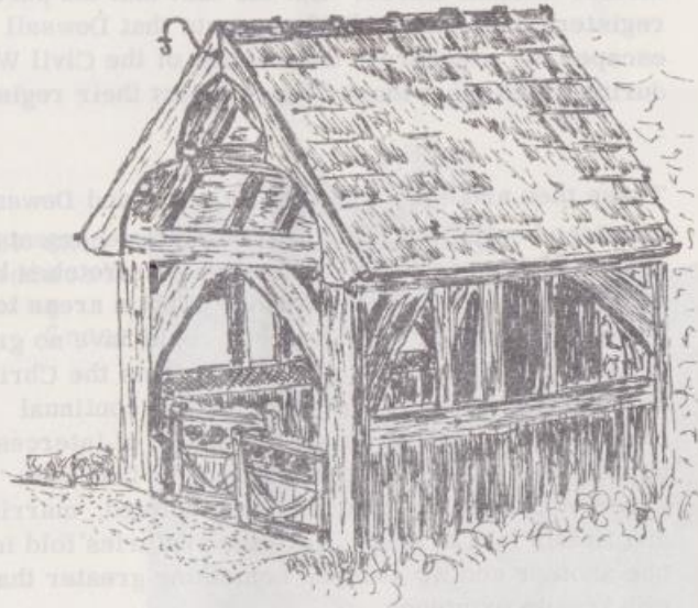
Dewsall South Porch
